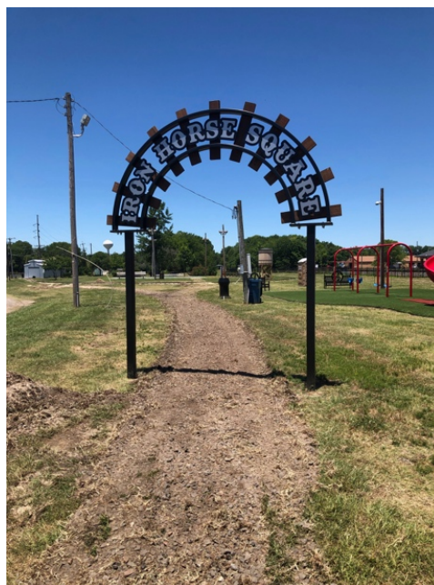
1 st day of work on walking trail.
